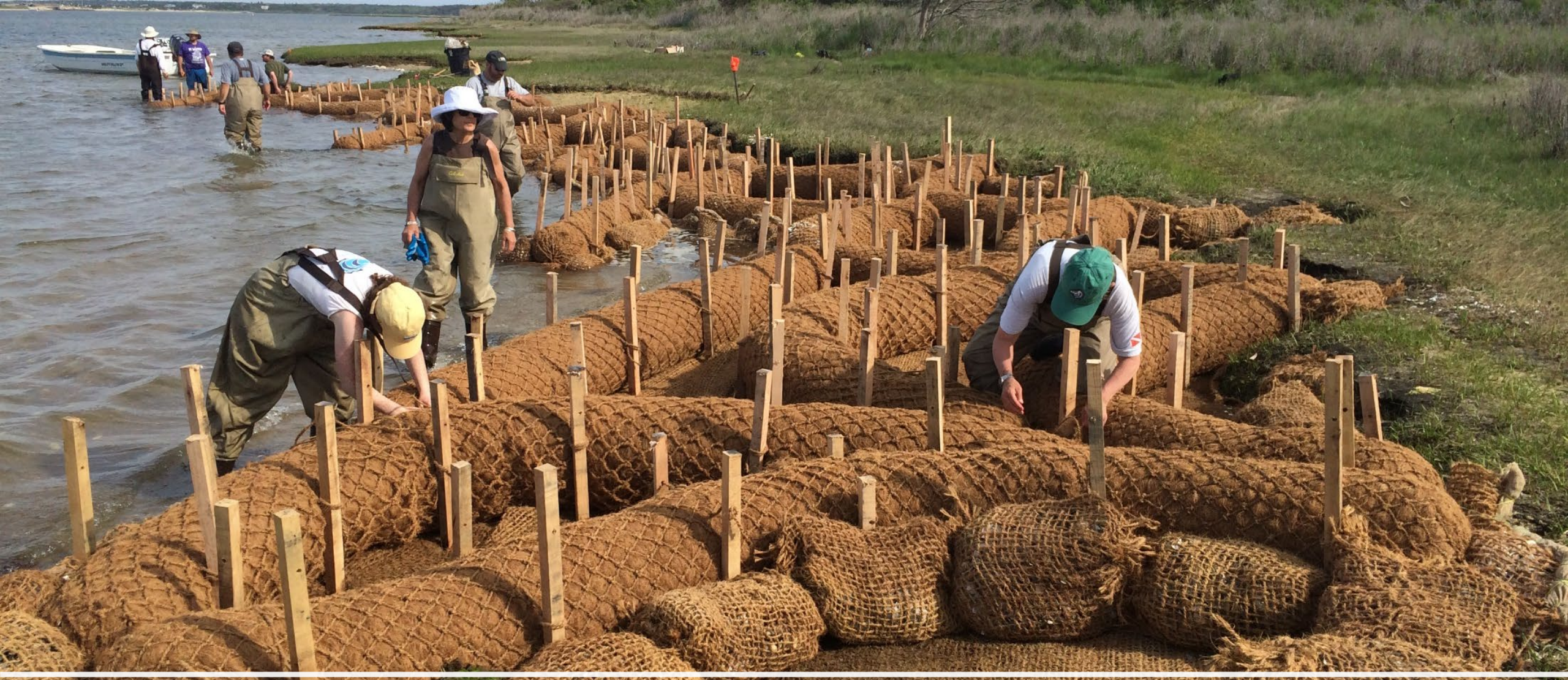
MV coir log installation
