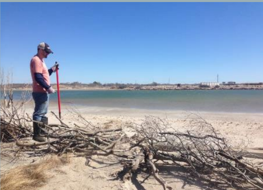
Used brush and dune fencing for sand stabilization
