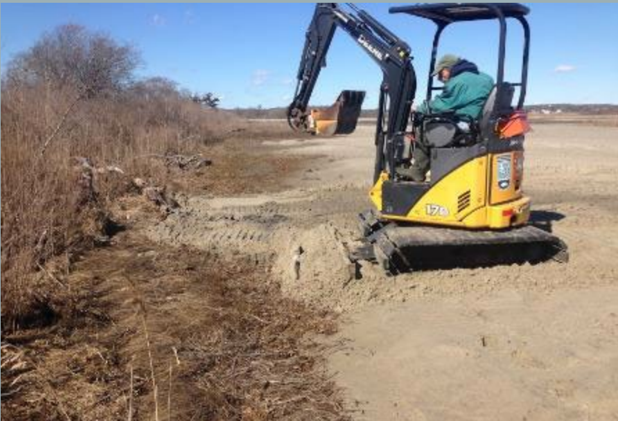
Regrading sediment to tie into existing elevations
