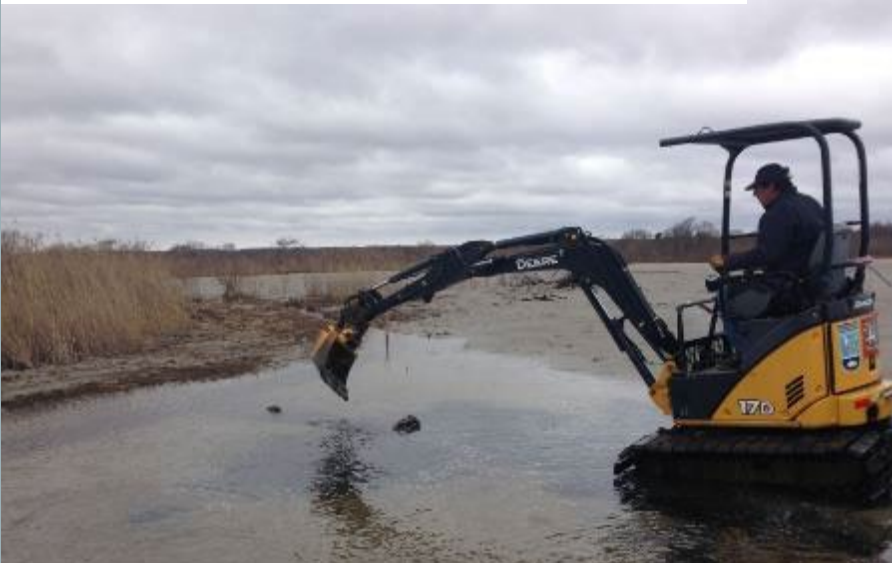
Impounded water along edge of sediment placement
